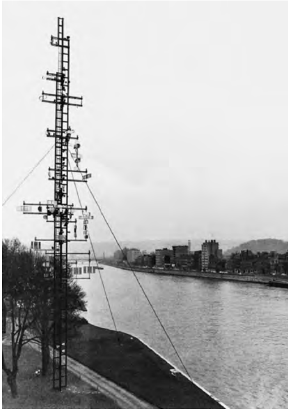
Nicolas Schöffer, Tower of Liège, installed next to the Congress Palace, Liège, Belgium, 1961.
